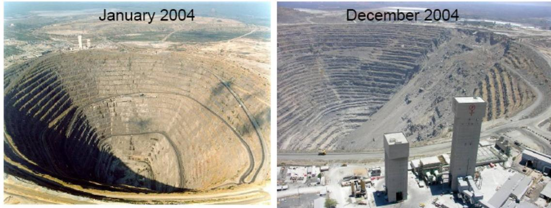
*Figure 2: Palabora Pit before and after failure*
