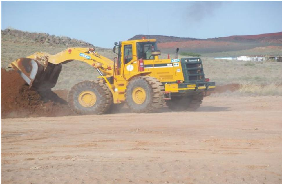
**Figure 6.3: Rehabilitation of earth dams in progress**
