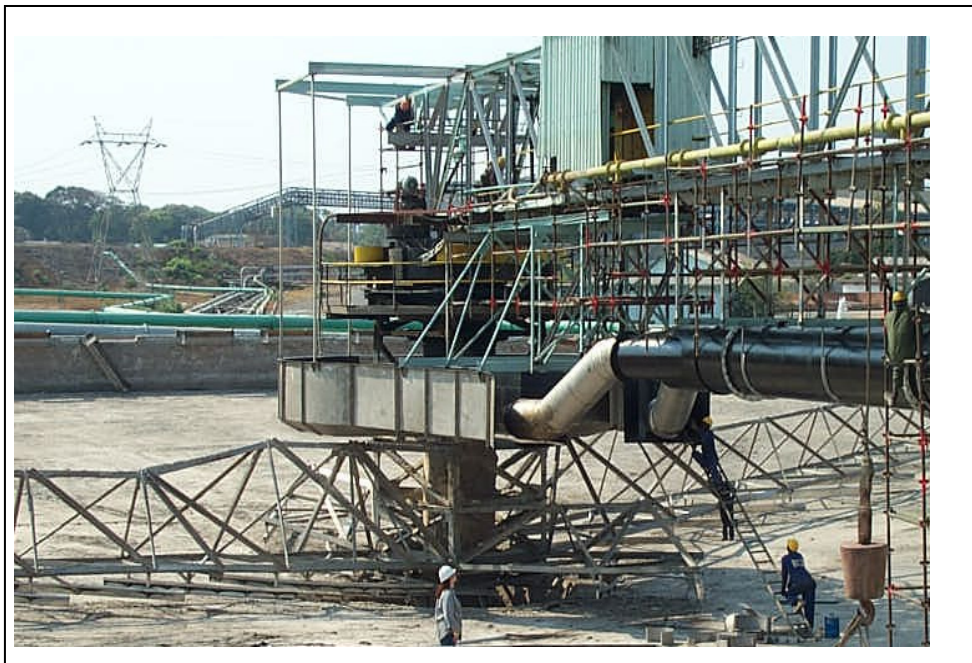
Fig 5. CCD 4 E-Duc installation works in progress.
